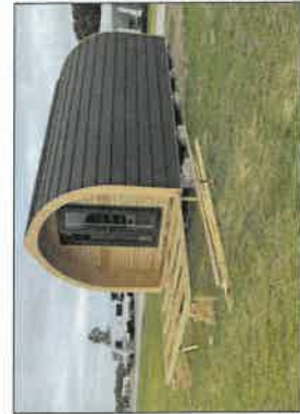
POD UNIT SUPPORTED BY TIMBER BEAMS RESTING UPON CONCRETE BLOCKS. TIMBER DECKING FIXED TO PARTLY BURIED POSTS
