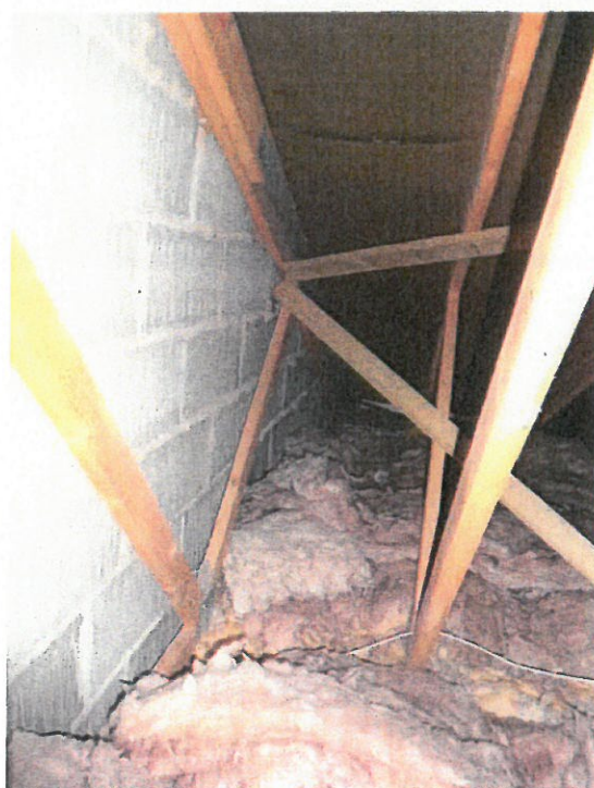
Photograph 12 – Lightweight concrete type block (Thermalite) internal skin to the extension
