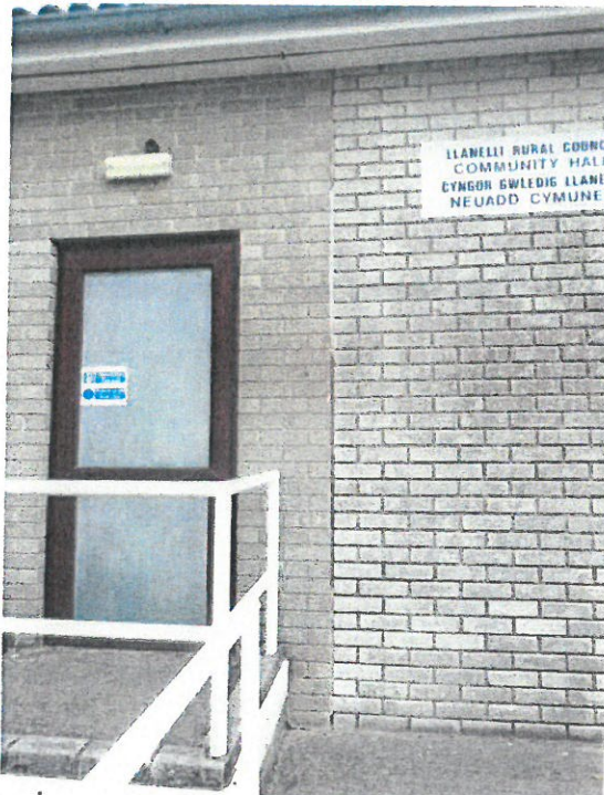
Photograph 8 – External expansion joint to front wall
