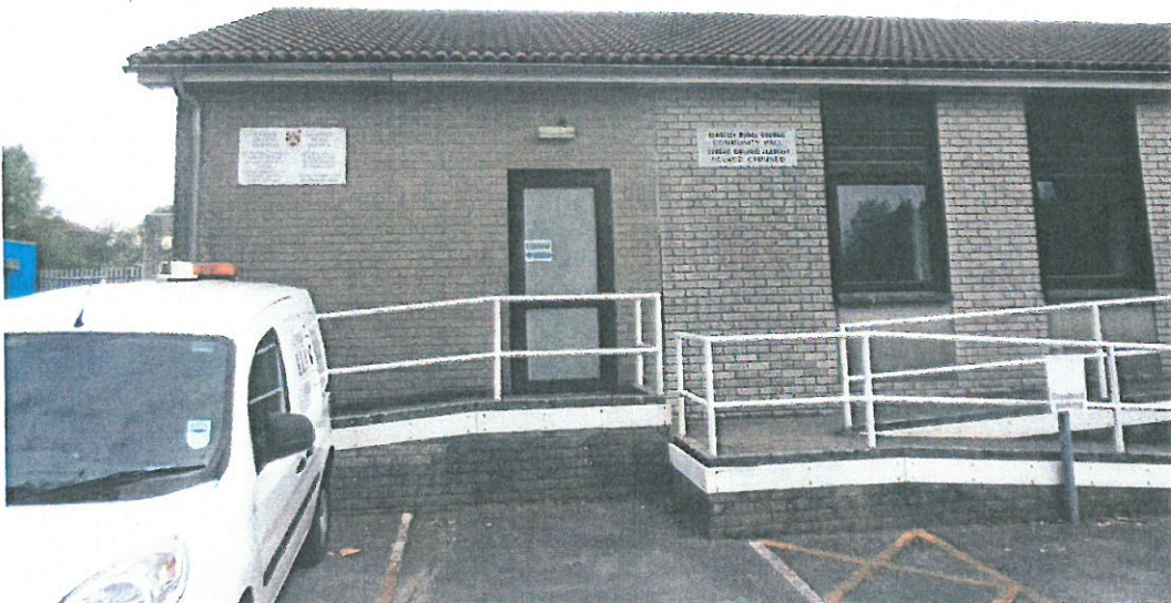
Photograph 10 – No signs of movement to roof
