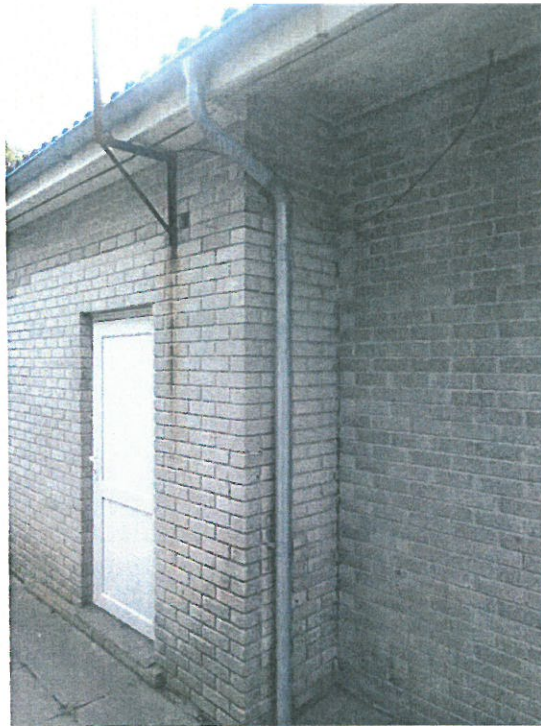
Photograph 9 – External expansion joint to rear wall
